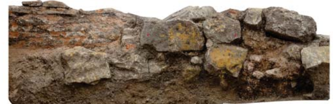
Relevé terme: praefurnium exterior
