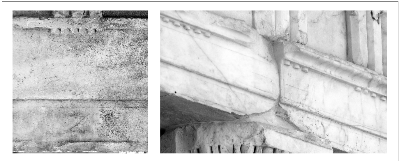
Fig. 7. The stonemason's mark on the short side of the architrave (left), detail of the architrave of the Aphrodisias Sebasteion South Portico.
