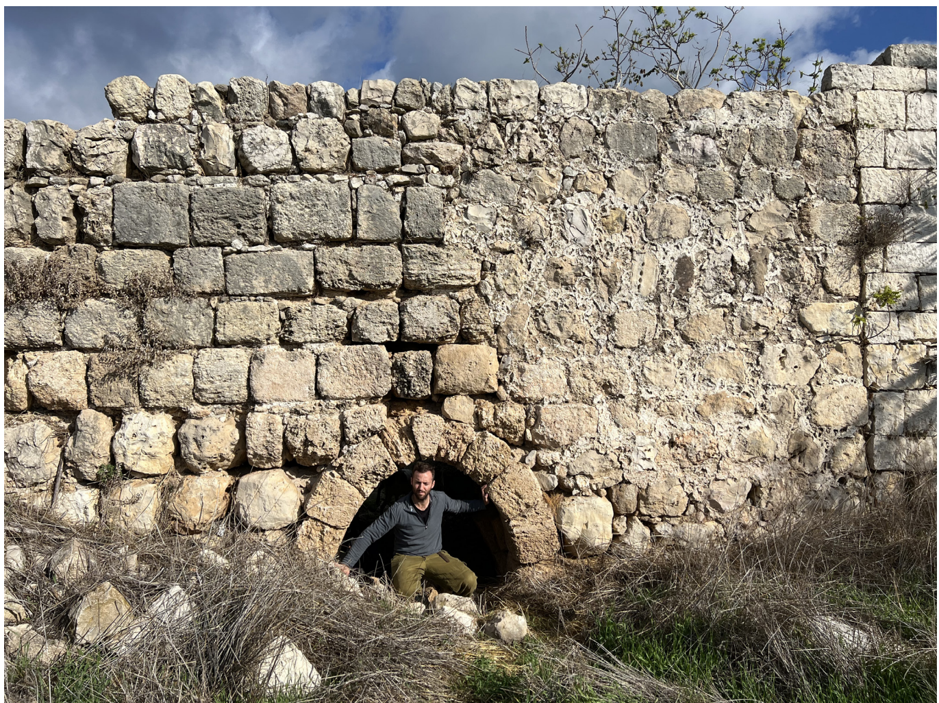
Fig. 8. Ground-floor entrance from the courtyard to a vaulted basement chamber below the hall house, looking north (B. Zissu).
