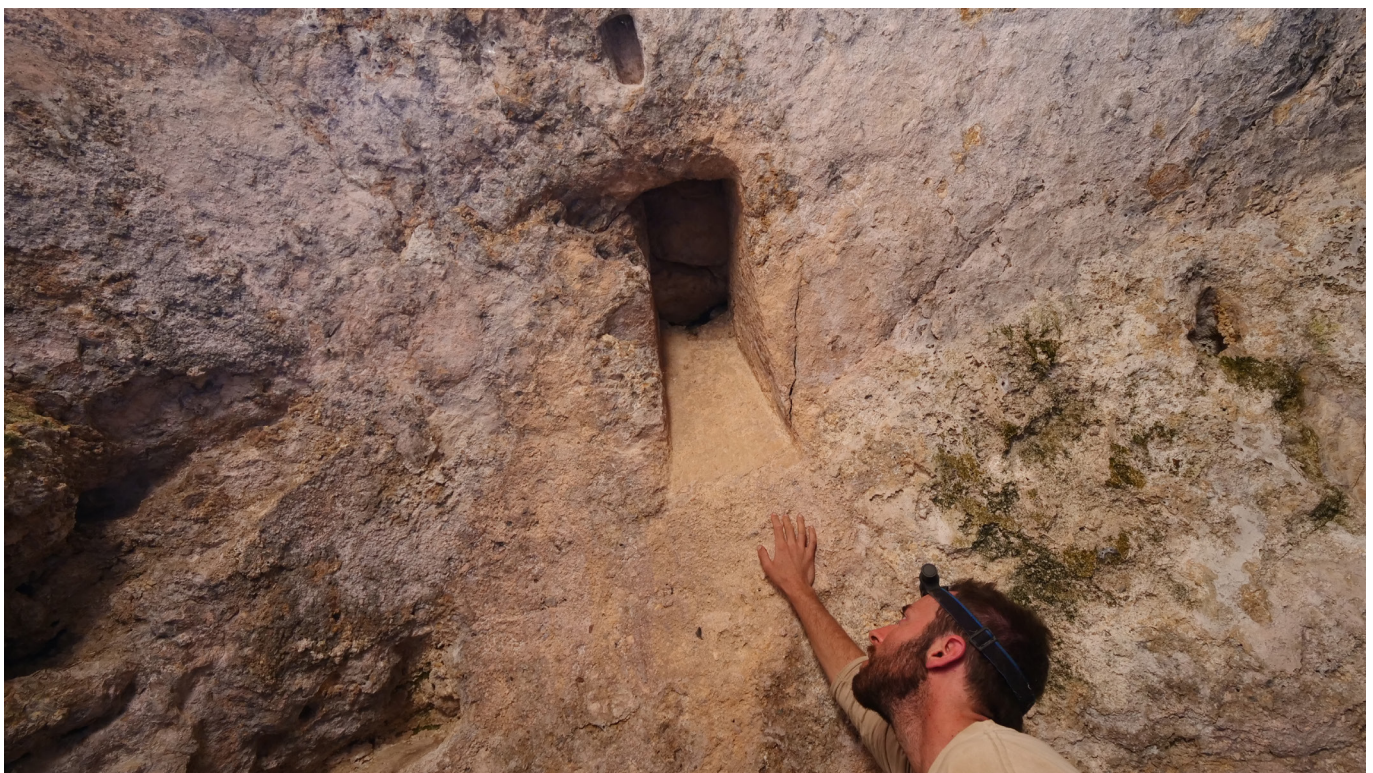
Fig. 22. Rock-cut details in the ceiling of cavity AT1.2 (B. Zissu).
